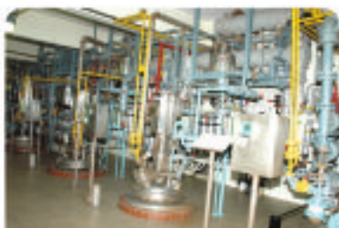
Pilot Plant - 13 Reactors
