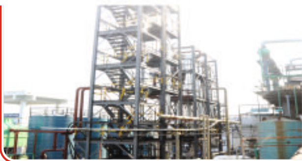
"Zero liquid discharge" facility
